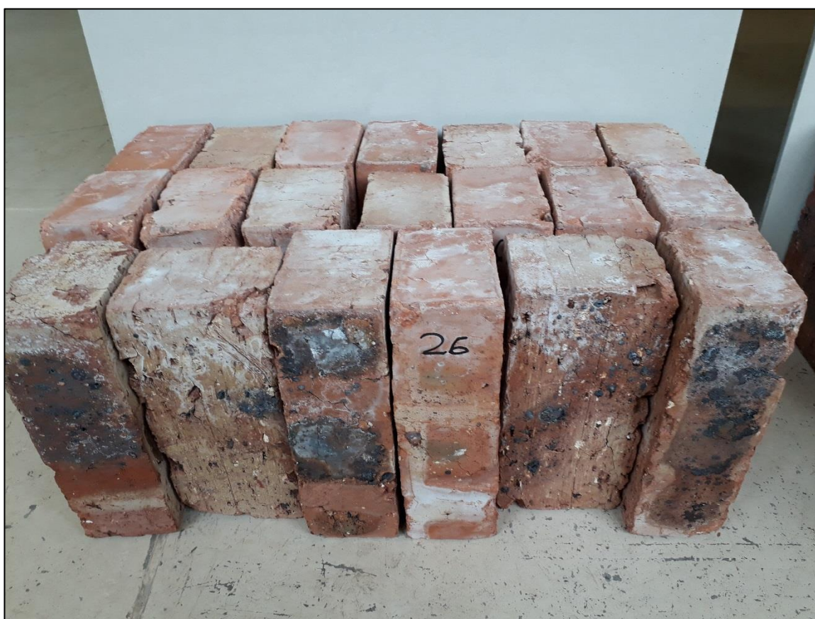
Figure 3.5.1: Samples after efflorescence testing
